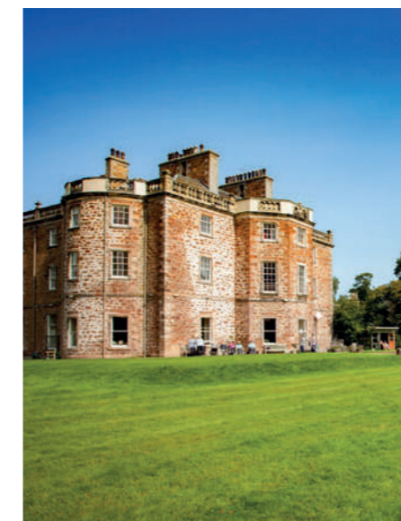
Leuchie House in East Lothian, Scotland, is a respite centre for people with multiple sclerosis. It is protected by an Advanced 4-loop MxPro 5 panel with AlarmCalm false alarm management.
