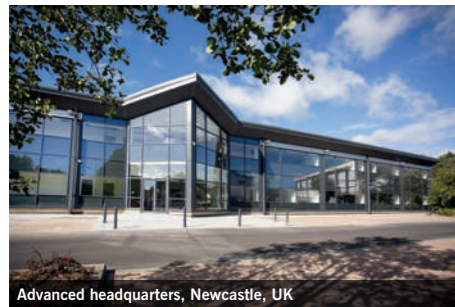
Advanced headquarters, Newcastle, UK
